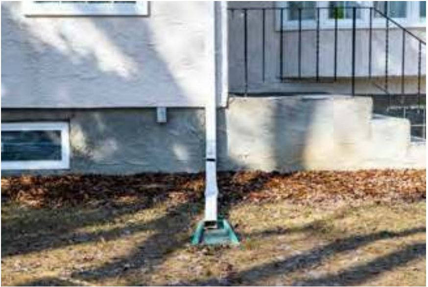
Photo: Splashpads help your yard absorb the water from your roof and protect against soil erosion.
