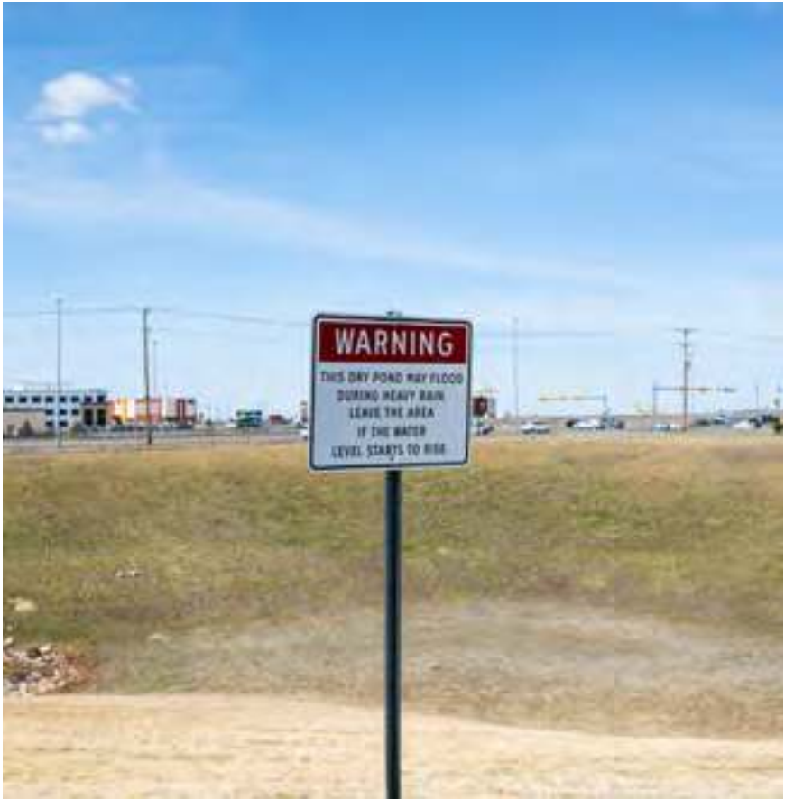
Photo: Dry ponds are designed to fill quickly during a heavy rain or quick spring melt.
