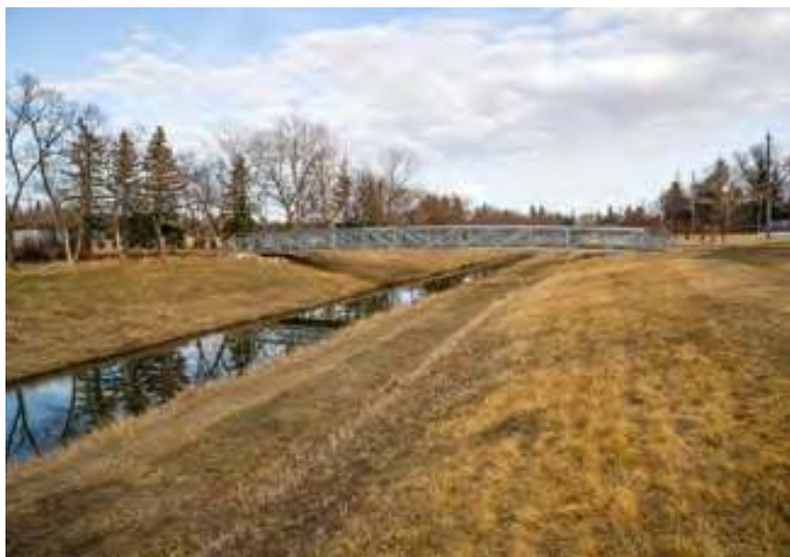
Photo: Drainage channels are part of the City's open space system.
