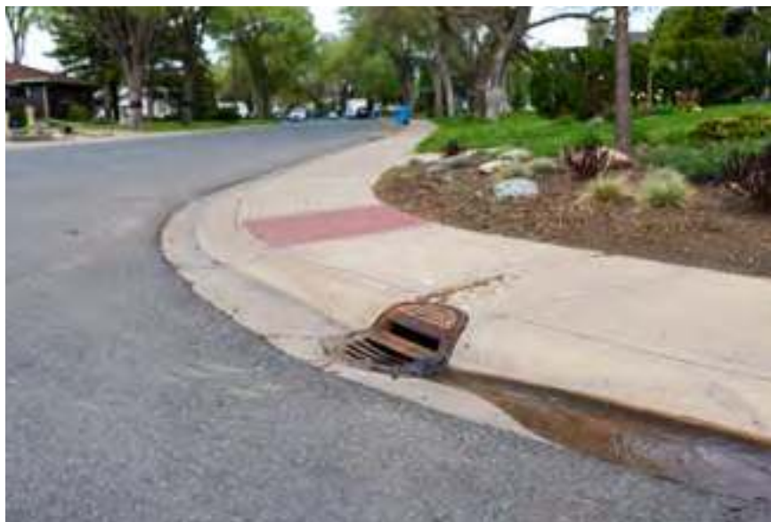
Photo: Entry points to the Public Drainage System are called Storm Drains.
