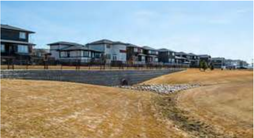
Photo: Dry ponds are often difficult to spot as they often pose as multipurpose sports fields.
