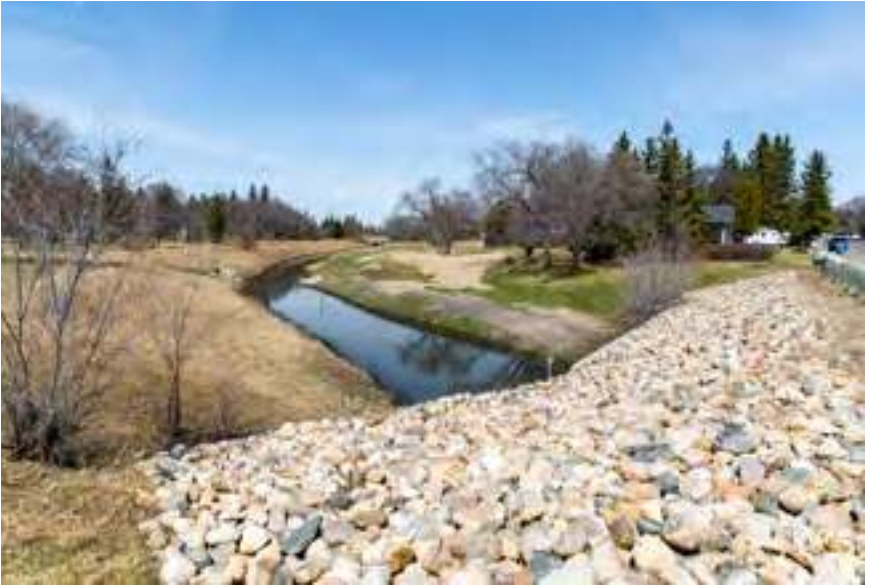
Photo: Drainage channels allow for large amounts of storm and melt water to be carried away into the natural system.
