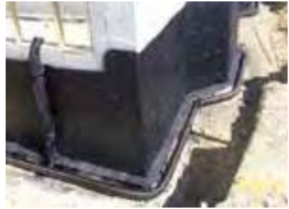
Photo: Weeping tile systems protect your basement and home from ground water. (Image Courtesy City of Edmonton)
